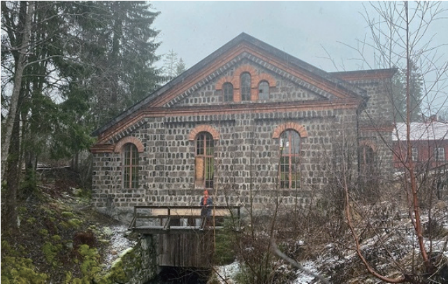
Fig.1 The waterpower plant in Hofors.
