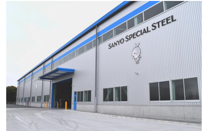
Product warehouse where solar power generation facility to be installed.
