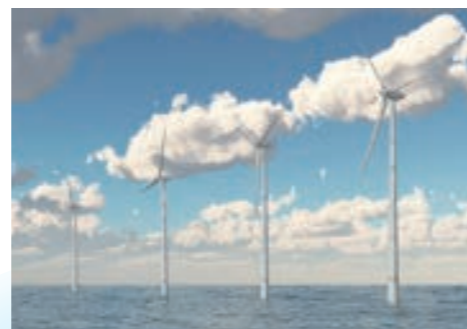
Fig. 1, A wind power generation facility
