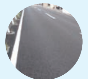
Recycled road paving in Himeji City
