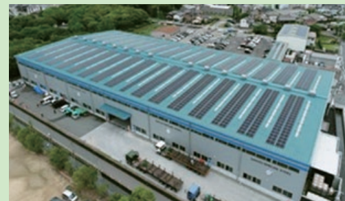
Solar power generation facilities on the rooftop of the product warehouse
