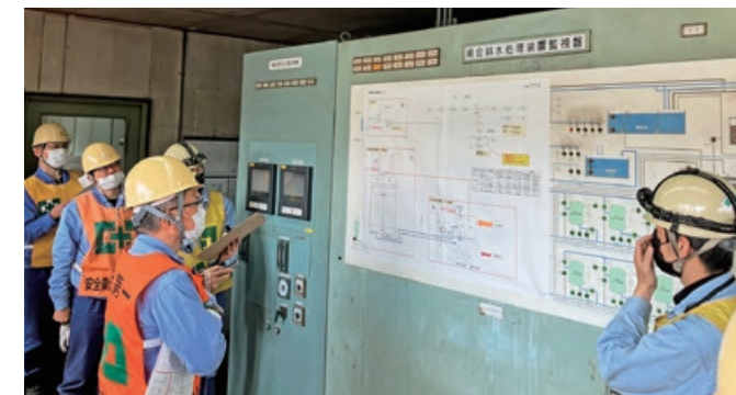
Patrol of wastewater treatment facilities
