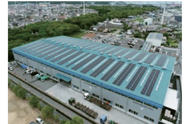
Solar power generation facilities on the rooftop of the product warehouse
